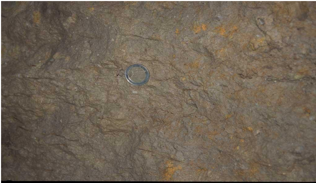
Figure 21-17: Mottling indicating periodic saturation due to a high water table (Photo: Donal Daly).
