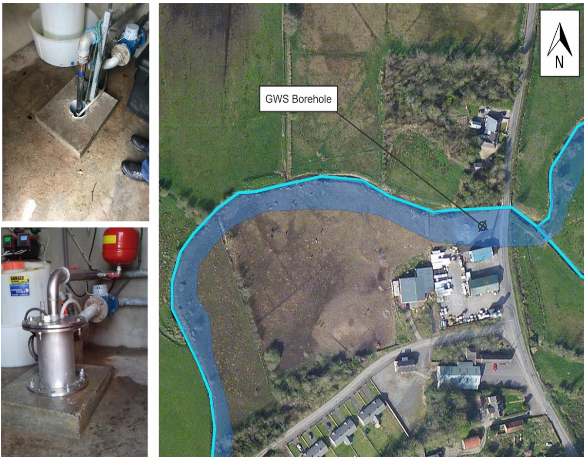
Figure 5a (Top Left). Borehole at Ballyallen GWS, Co. Carlow. Figure 5b (Bottom Left). Borehole at Ballyallen GWS, post well head improvement works. Figure 6. (Right). Location of Templeport GWS’s abstraction borehole within potential fluvial flood zone (i.e. blue hatch is indicative of the 1 in 100-year fluvial flood zone predicated during the Preliminary Flood Risk Assessment (2011)).
