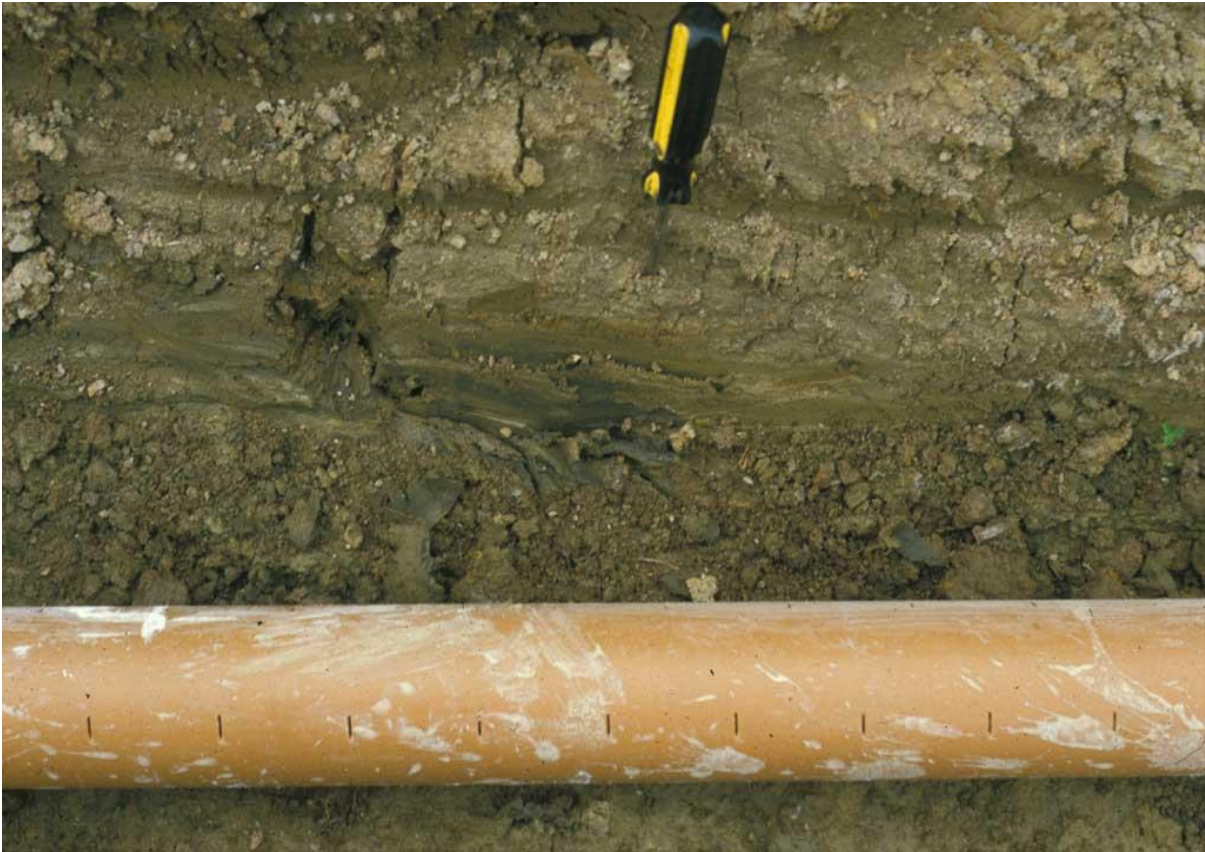
Figure 21-6: Grey, low permeability subsoil. Note 'plasticine' nature of the subsoil. (Photo: Donal Daly)
