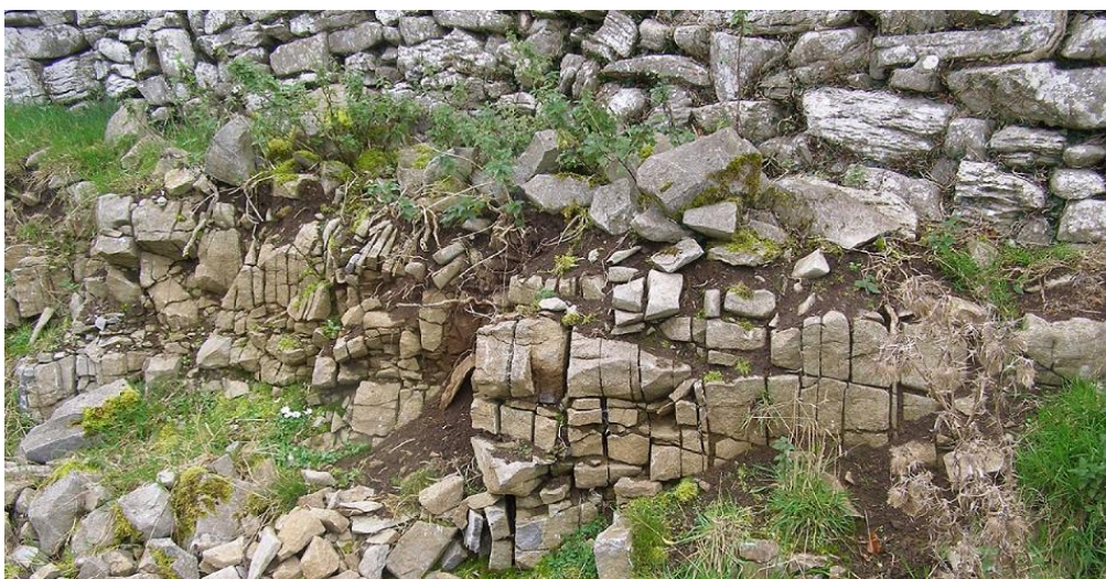
Figure 10-19: Joints in limestone (Photo: Donal Daly).
