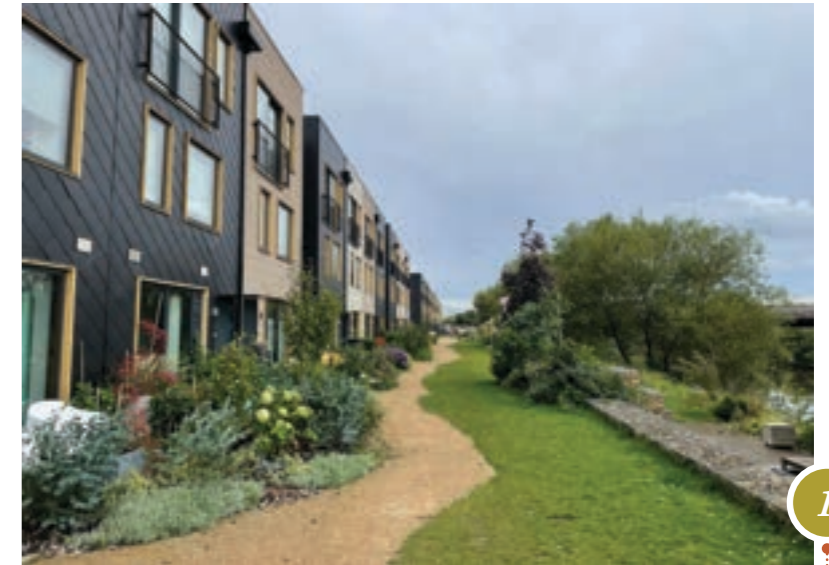
Figure 6: Filter Drain - Climate Innovation District, Leeds
