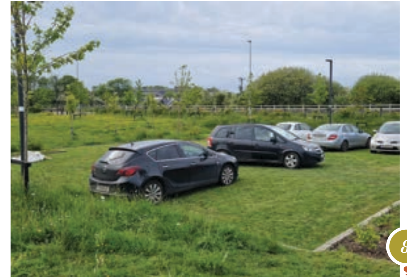
Figure 20: Proprietary Reinforced Grass - Min Ryan Park, Wexford
