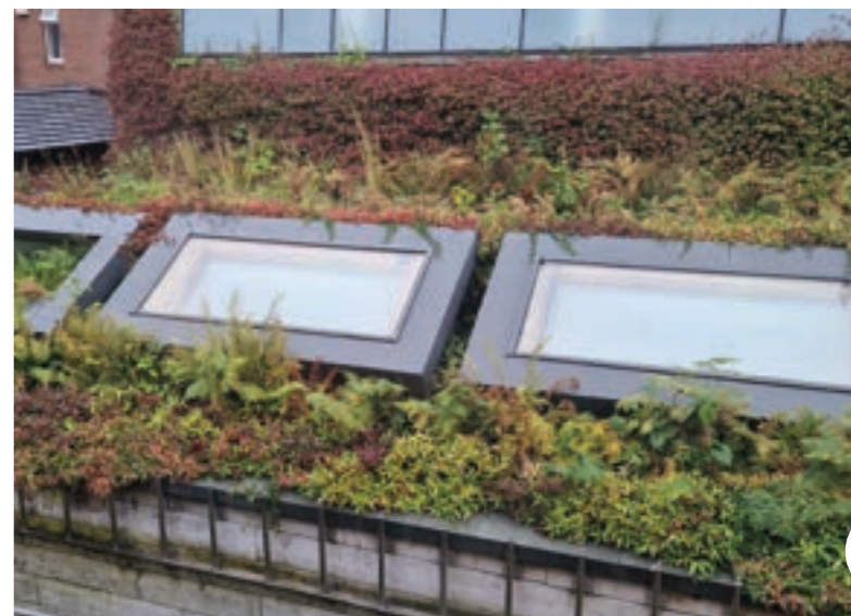
Figure 18: Green Roof - Engineers Ireland, Clyde Road, Dublin
