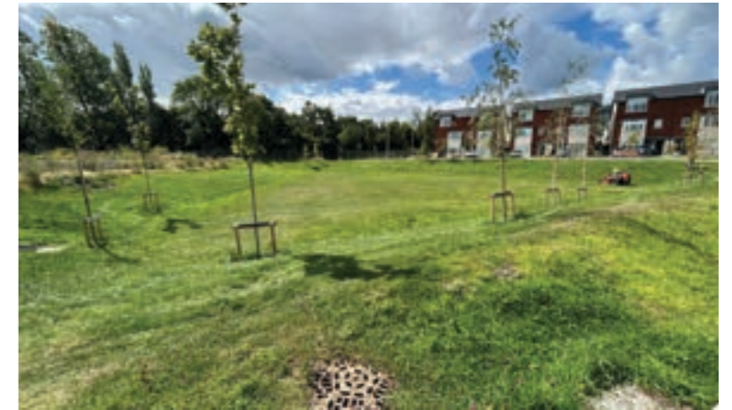
Figure 25: Detention Basin – Kilgobbin, Dublin
