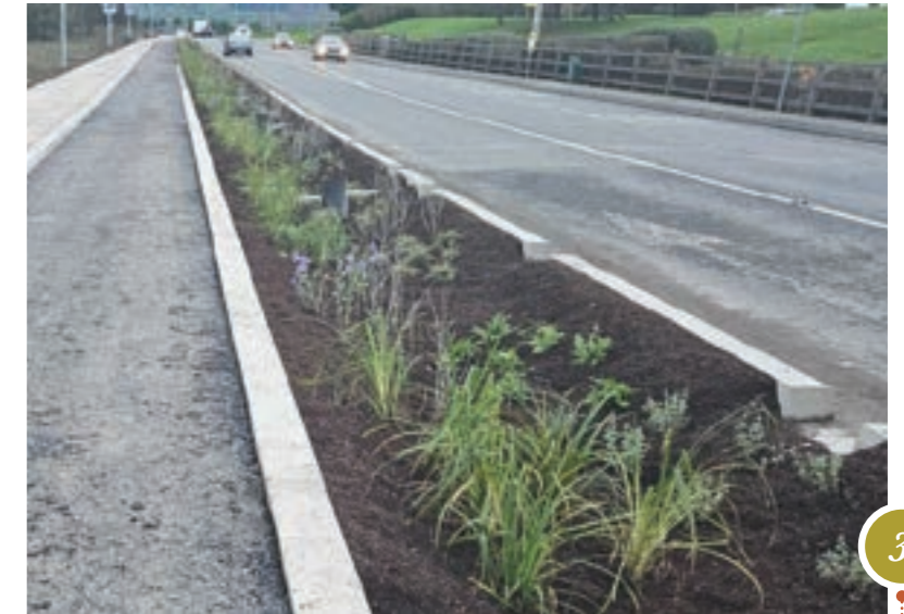
Figure 10: Linear Raingarden - Cashel Road Active Travel Scheme, Clonmel, County Tipperary
