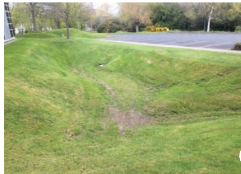
Figure 14: Detention Basin - City West, Dublin
